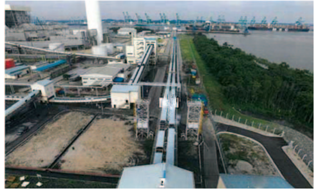
Detailed design of a new coal import conveying system for a power station in Malaysia included the upgrade of the existing grab-type ship-unloader (above, left) and adding a new conveying stream from the import jetty to the existing power station stockyard facility (above, right).
