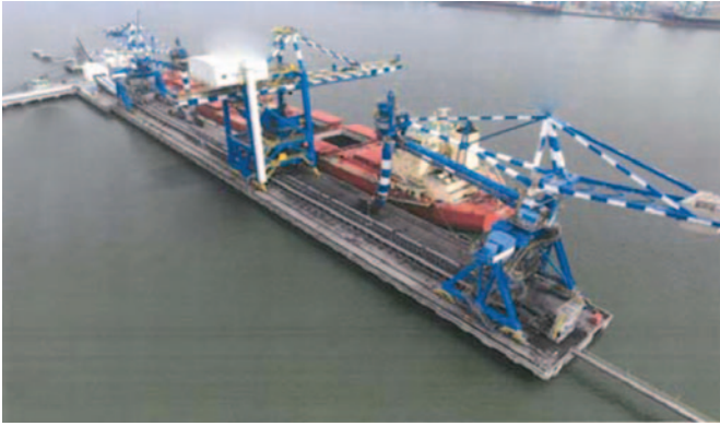
Detailed design of a new coal import conveying system for a power station in Malaysia included the upgrade of the existing grab-type ship-unloader (above, left) and adding a new conveying stream from the import jetty to the existing power station stockyard facility (above, right).
