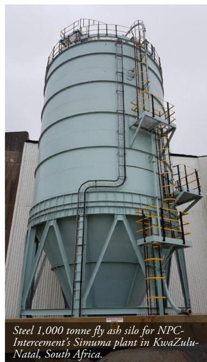
Steel 1,000 tonne fly ash silo for NPC-Intercement’s Simuma plant in KwaZulu-Natal, South Africa.
