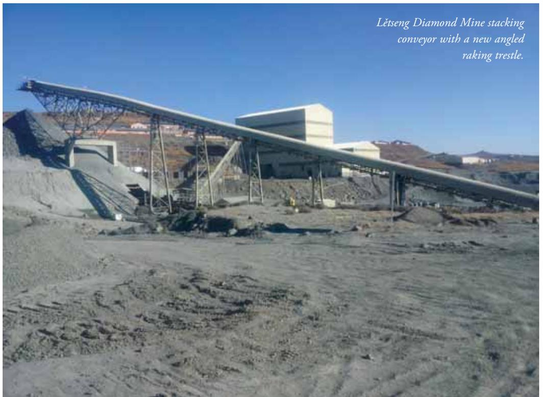
*Letšeng Diamond Mine stacking conveyor with a new angled raking trestle.*
