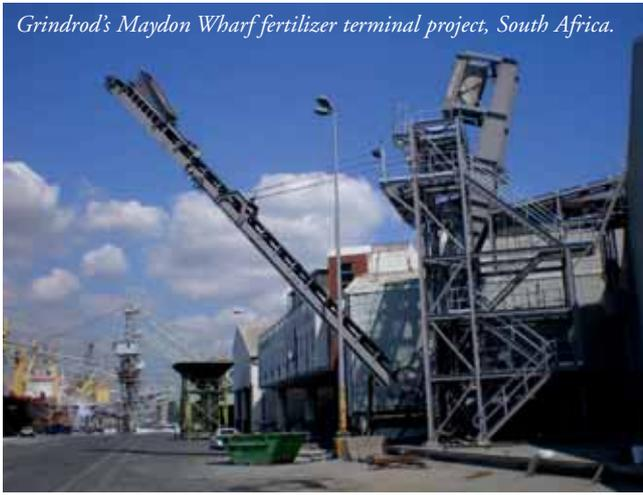
mounted conveyors stationed on the jetty at locations to suit the ship docking arrangements. Once the ships have been offloaded, the fertilizer is conveyed to a central pivoting and retractable boom conveyor.
